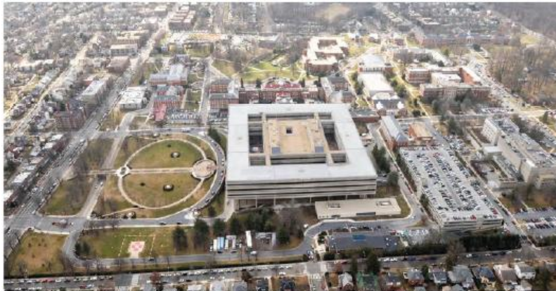
Figure 8-199: Aerial photograph of Walter Reed campus looking south with Building 2 in the foreground. (BEFORE) Source: WRAMC Base Transition Coordination Office
