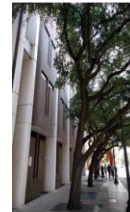
Bldg R - Market
