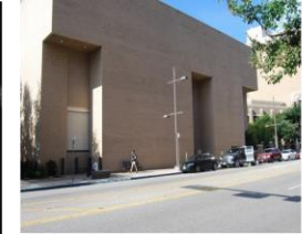
Bldg C - Main
