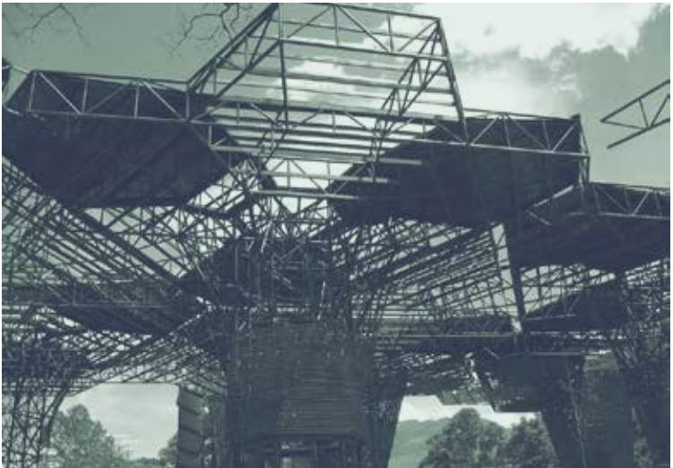
Figure 97| The canopy formed by the petals filters light at the same time that collects rainwater for watering plants.
