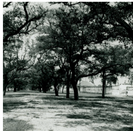
North Claiborne neutral ground before construction. (WWNO)
