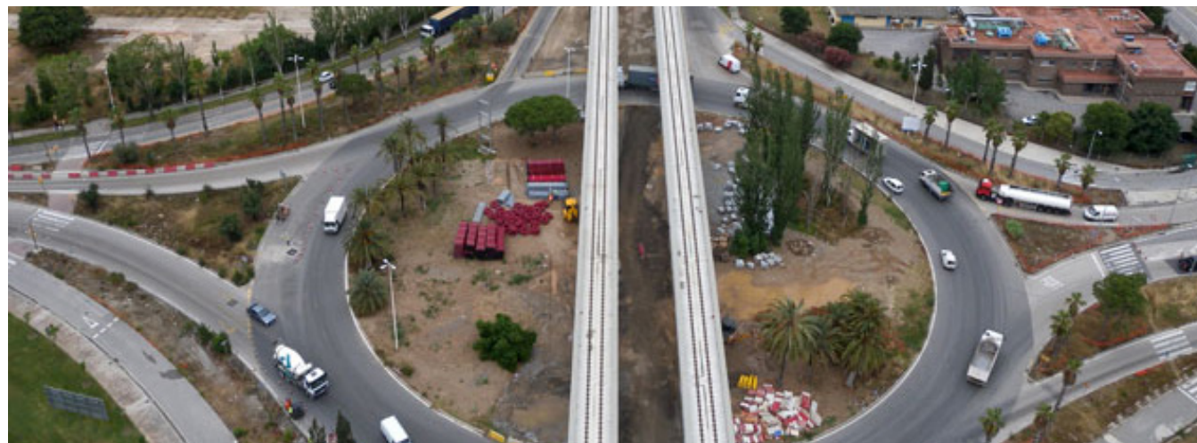
Roundabout intersections on Street A contain large green spaces. The street is still under construction in this image. (Pacadar)
