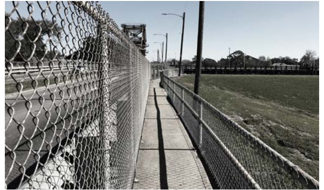
B Aerial View looking over Claiborne Bridge
