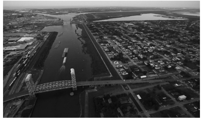
B Aerial View looking over Claiborne Bridge
