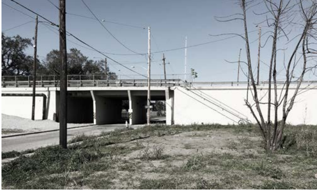
C View of St. Claude Bridge on Pedestrian Walkway
