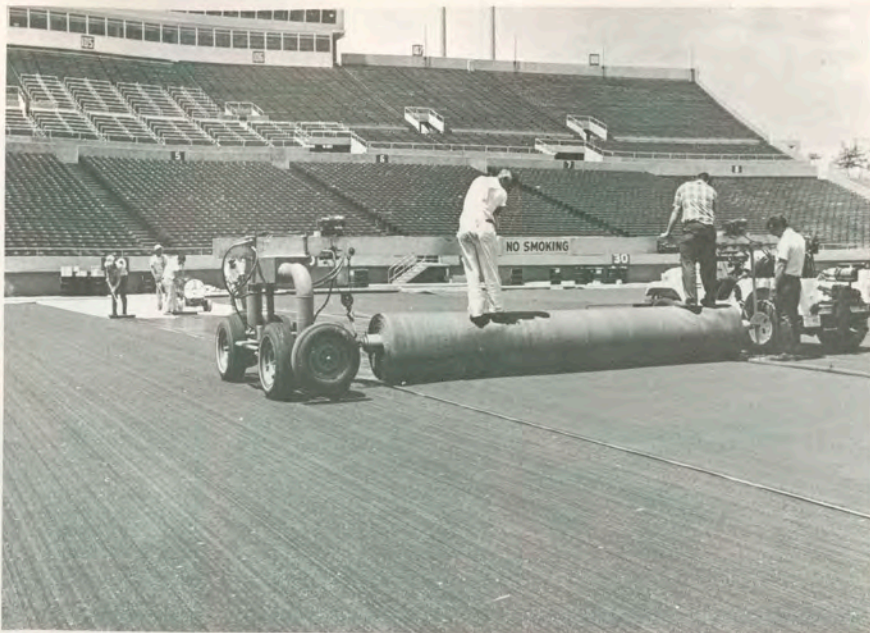
The AstroTurf is laid in alternating strips atop the foam rubber padding. Heavy glue cements the synthetic turf to the pad.
