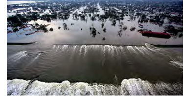
New Orleans levee breach during Hurricane Katrina [via http://www.hurricanekatrina.com ]
