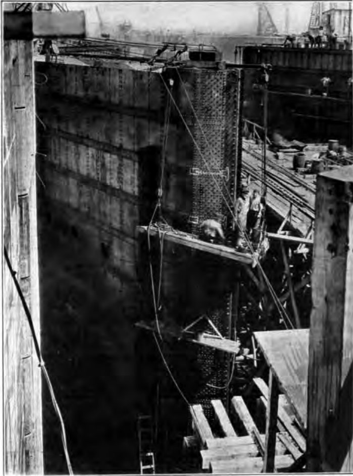
View of the Lock Gate
