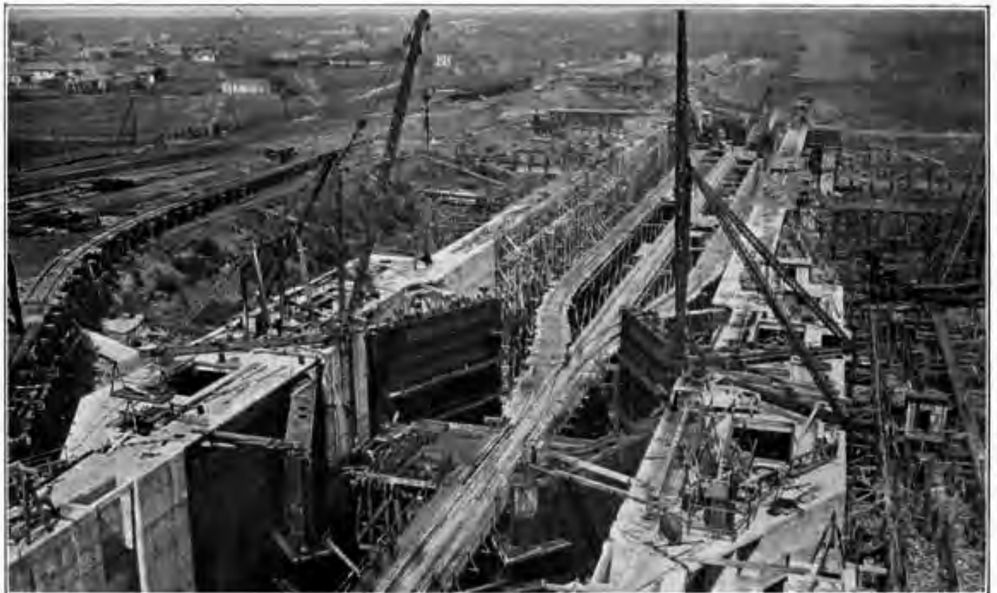
View While Building the Lock
