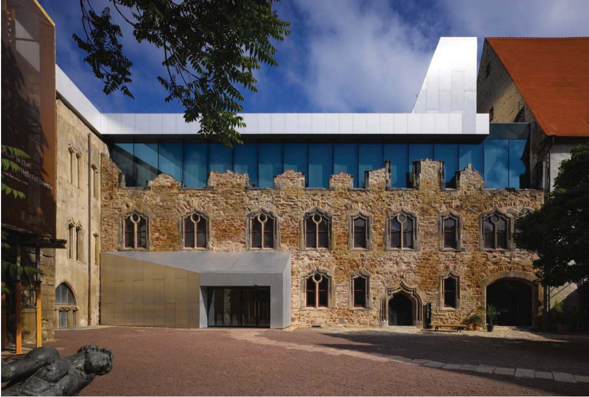
Fig. 25. Facade. New sits behind old
