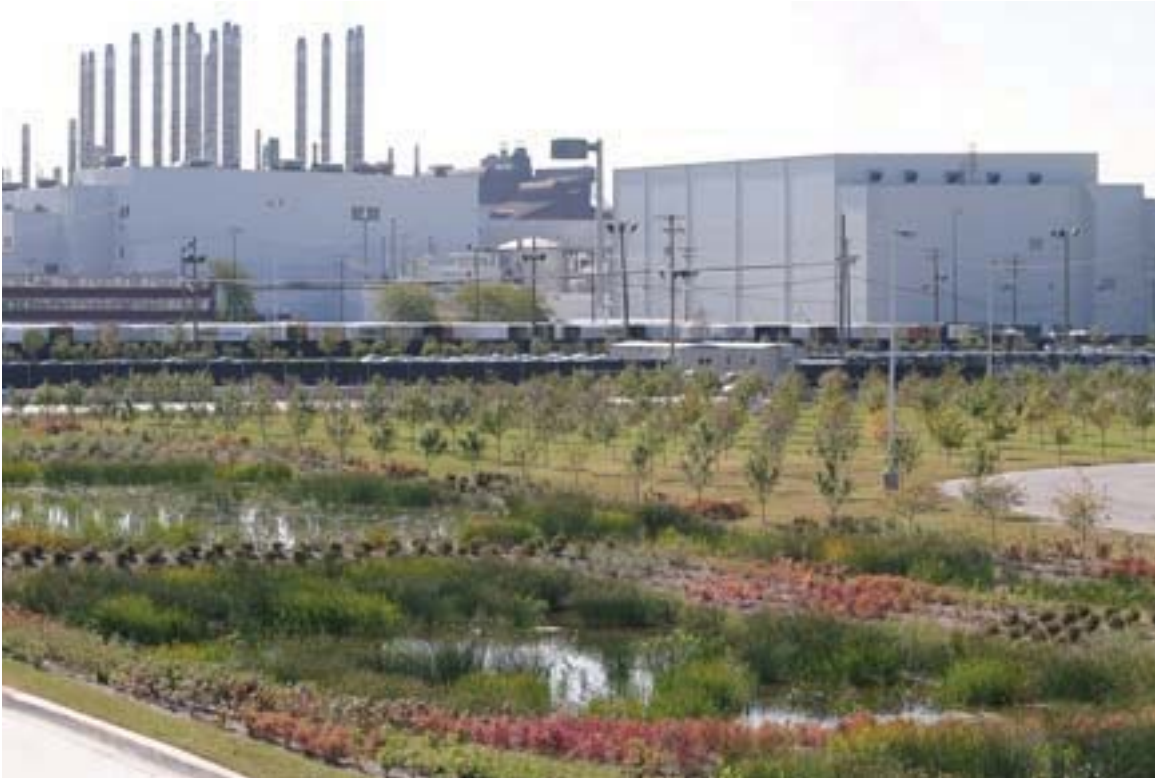
Fig. 20. View of water retention landscape
