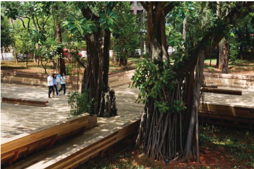
Fig. 23. Deck is elevated with steel structure
