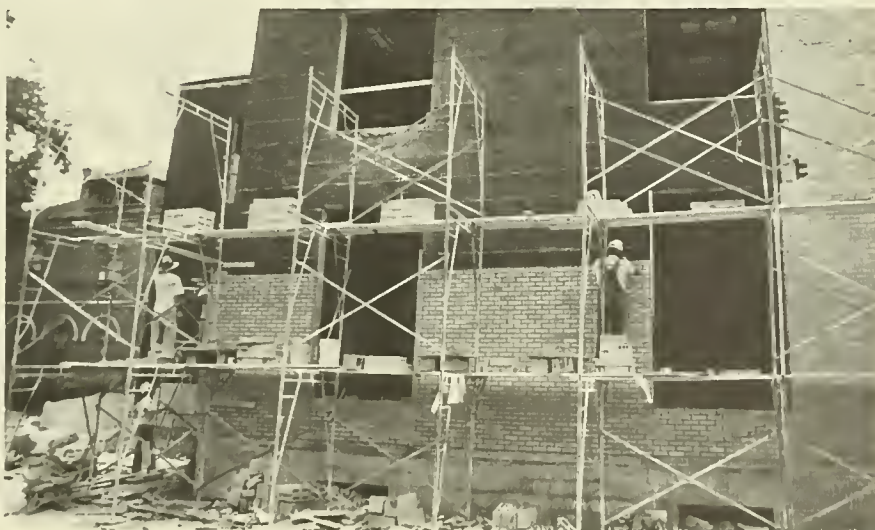
CONSTRUCTION ON Hebert Hall continues long past the scheduled completion date.
