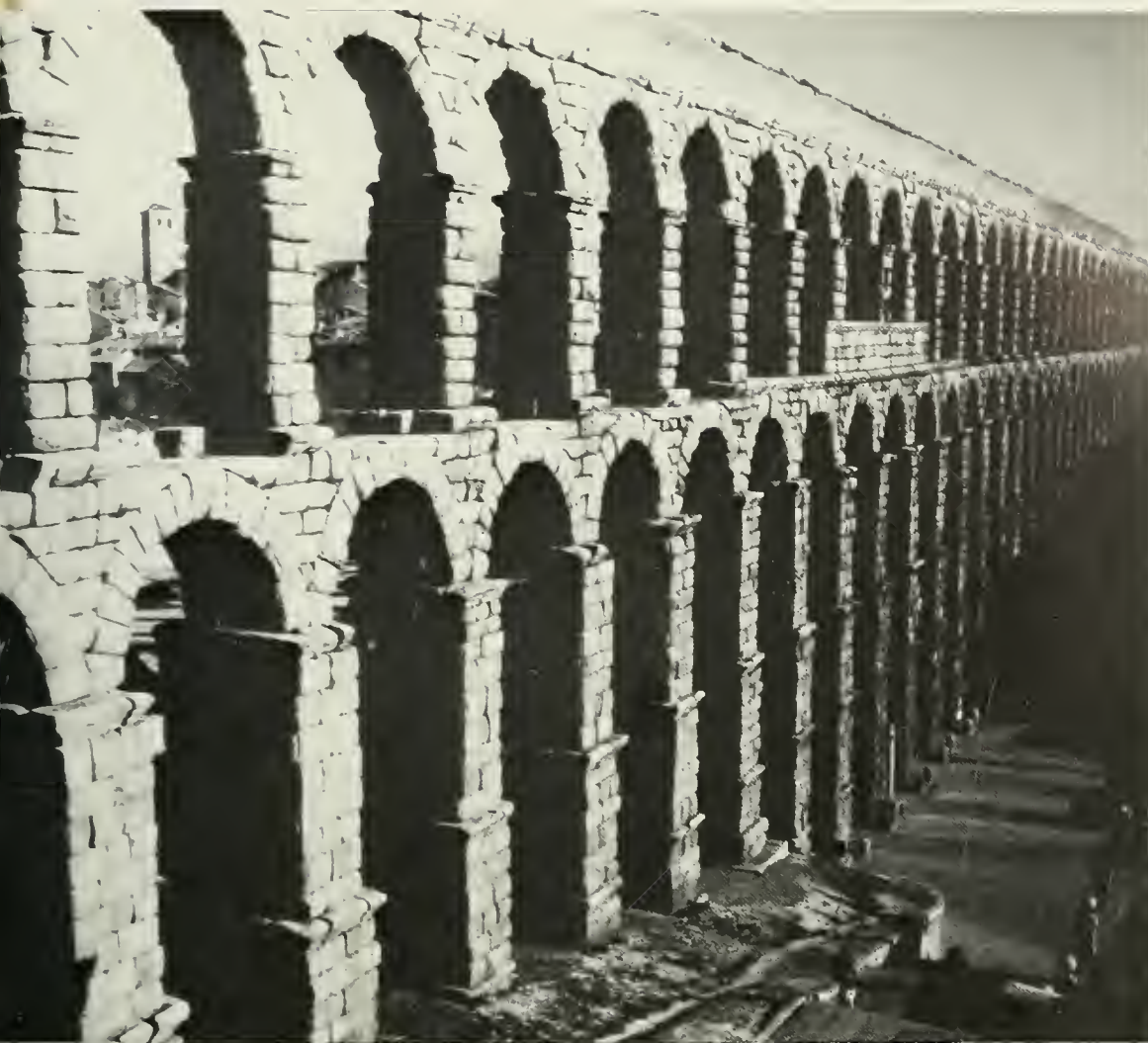
The Roman Aqueducts in Segovia, Spain are not only standing, but still in use.
