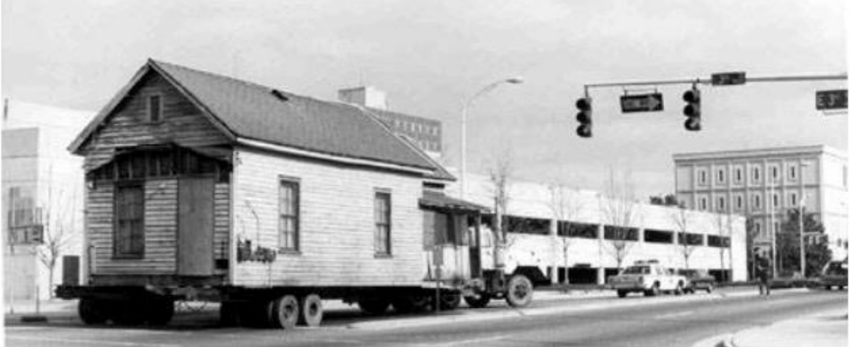
Shotgun house en route to its new location
