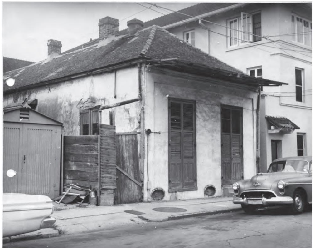
Figure 16a. The Helen LePage Maisonette, 1024 Gov. Nicholls Street, Square 106, Vieux Carré. Courtesy Hilary Irvin, New Orleans Vieux Carré Commission. The house is extant and may well be the oldest surviving shotgun-type house in New Orleans and the nation. It was constructed by the Haitian immigrant Pierre Roup in 1823, beside his own shotgun maisonette residence (Ref. NONA Felix de Armas [notary] March 17, 1836: 104:35).
