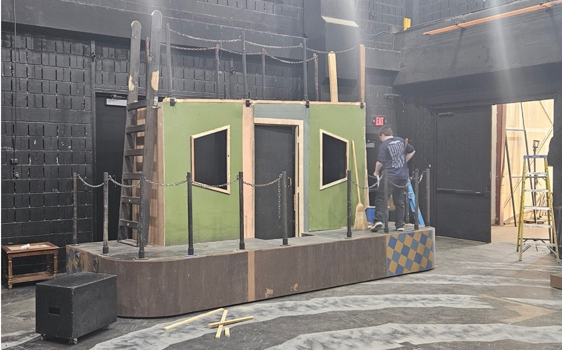
Figure 36: Louks, Kaeanne. Image of the faced houseboat in the Lupin Theatre, complete with door, window openings with frames, ladders, and most of the railings. In the background, the doorway between the scene shop and the theater can be seen. 2024, Tulane University.
