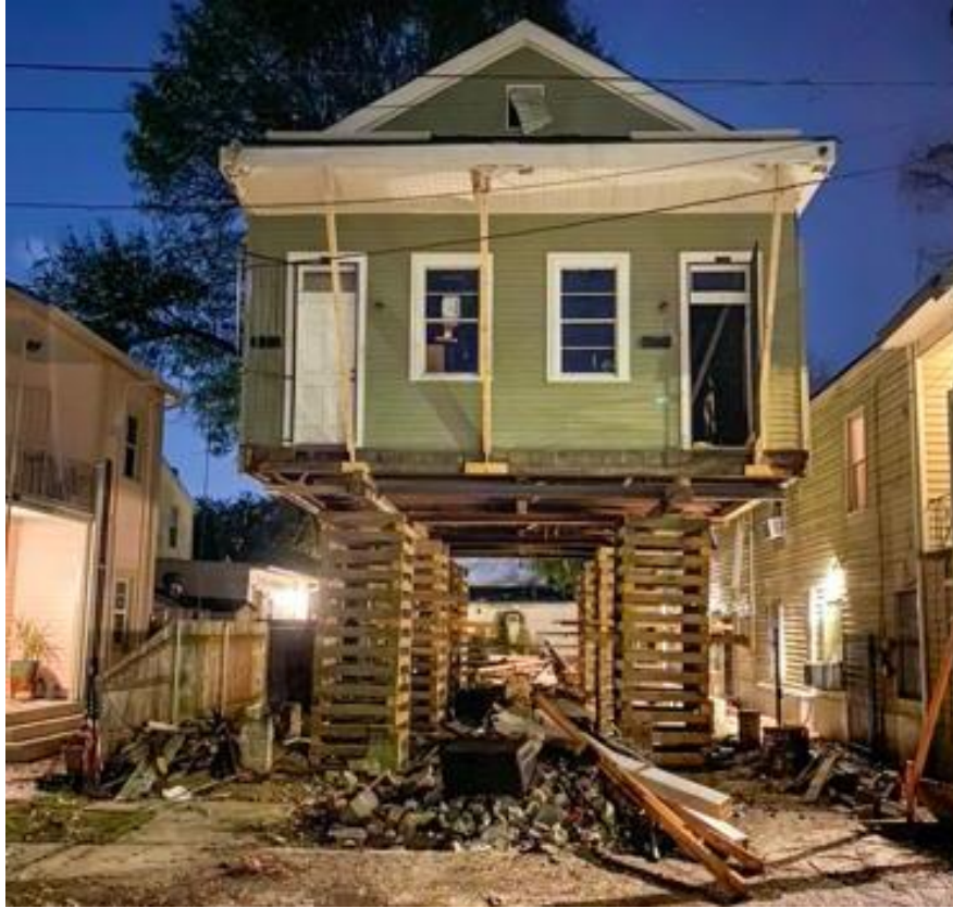
Figure 23: Raised up double shotgun to create a dormitory type of residence. Photo by David Grunfeld. “We’re Fed Up’: Uptown Homeowners Say ‘Doubles to Dorms’ Replacing Longtime Residents with Students.” The Times-Picayune , October 5, 2022. https://www.nola.com/news/business/article_86abdaf0-4366-11ed-a6d2-8b243904731f.html .
