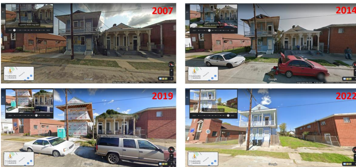
Renovation, demolition, and new construction from 2007-2022 (2005-21 First Street, New Orleans, LA 70113)
