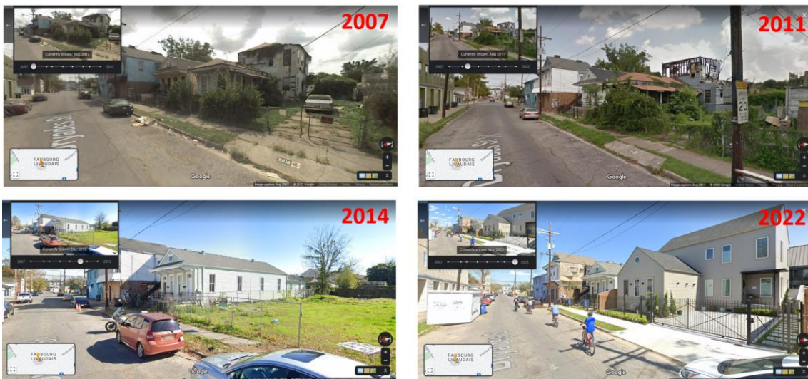
Demolition and new construction from 2007-2022 (2514-18 Dryades Street, New Orleans, LA 70113)
