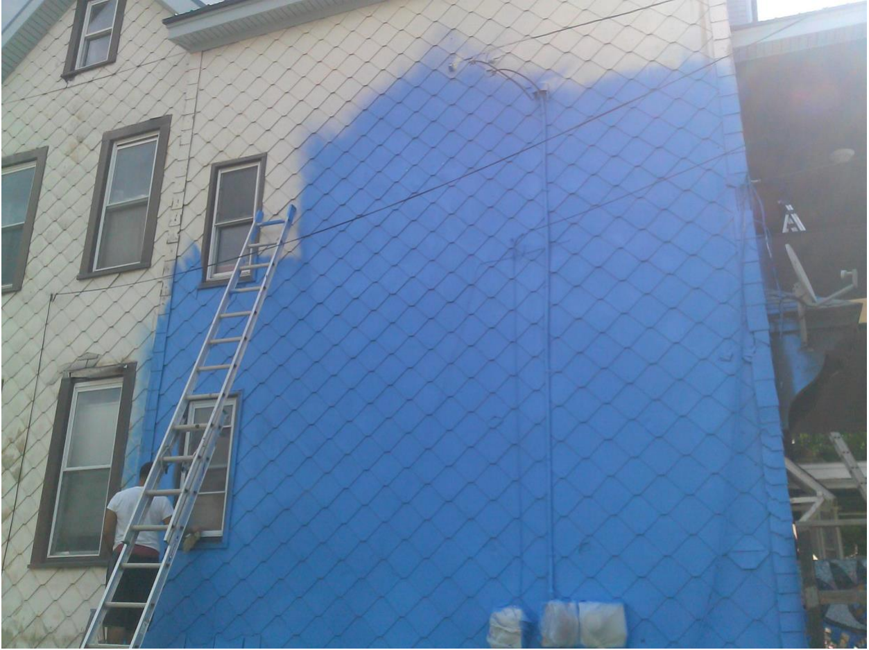
Figure 15: Image of ARThouse under construction. Courtesy of Love Front Porch, 2015
