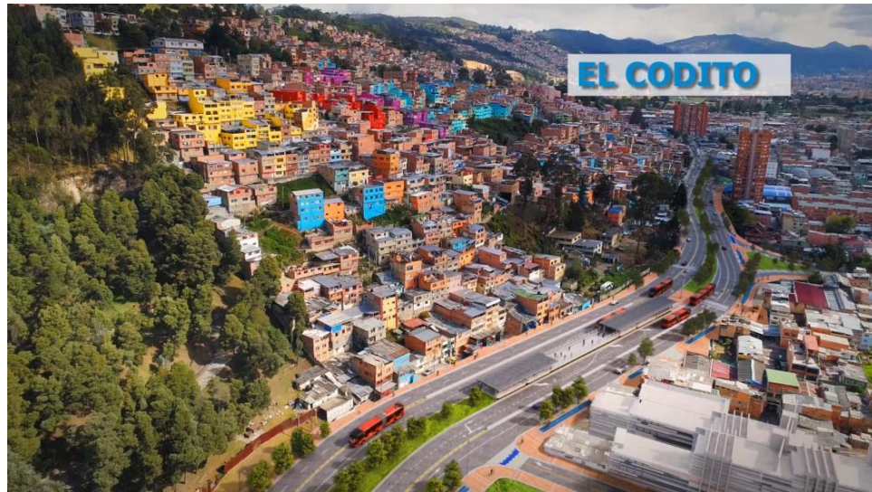
Figure 13: Projected TransMilenio trunk line on Carrera Séptima in the north of Bogotá (image from city government website—Maldonado 2019)
