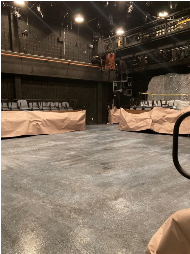
Figure 91 (Above): The floor is base-coated. 2021, Tulane University.
