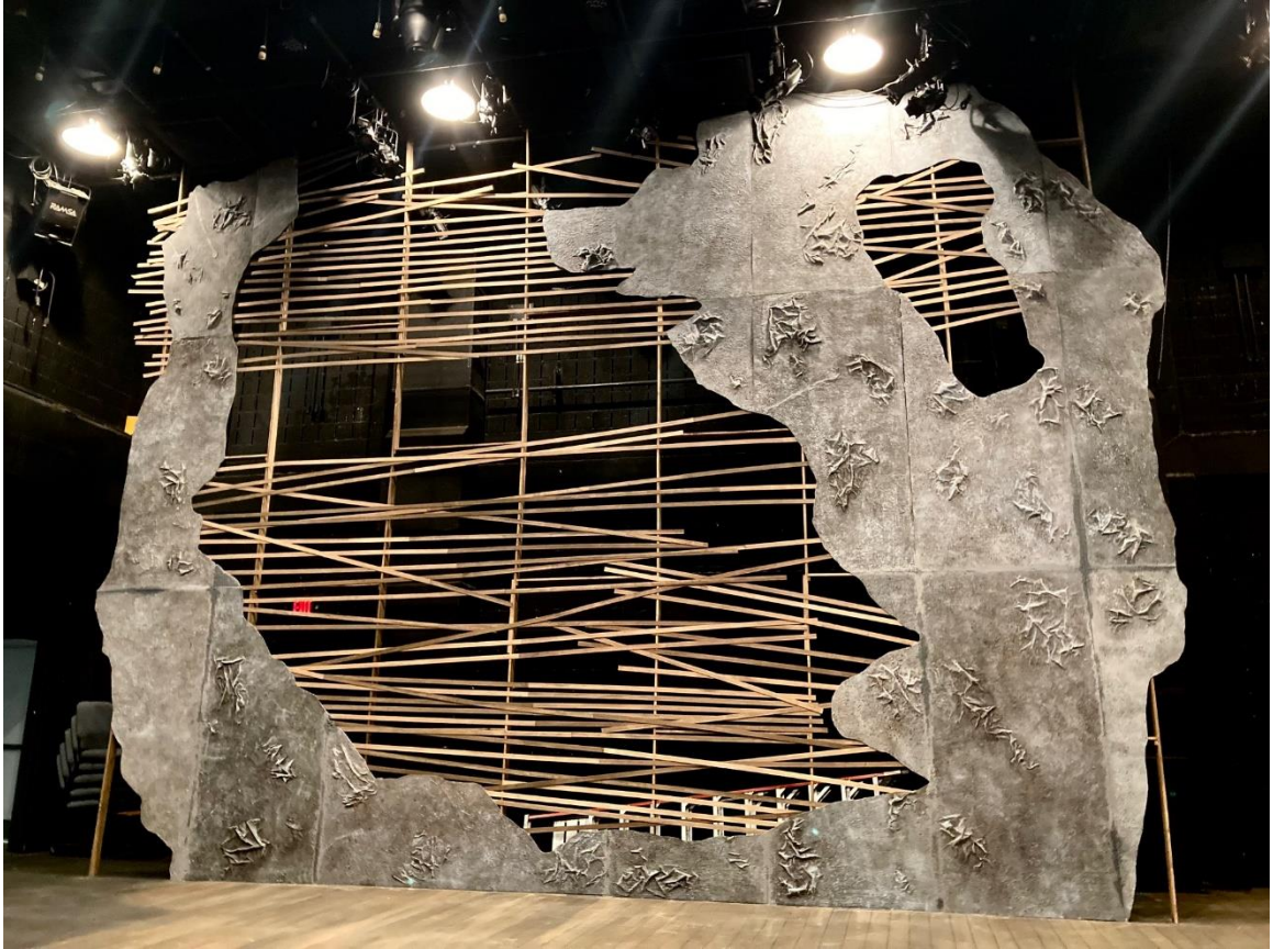
Figure 74: Assembly of the wall is complete except for some slats in the upper third. 2021, Tulane University.
