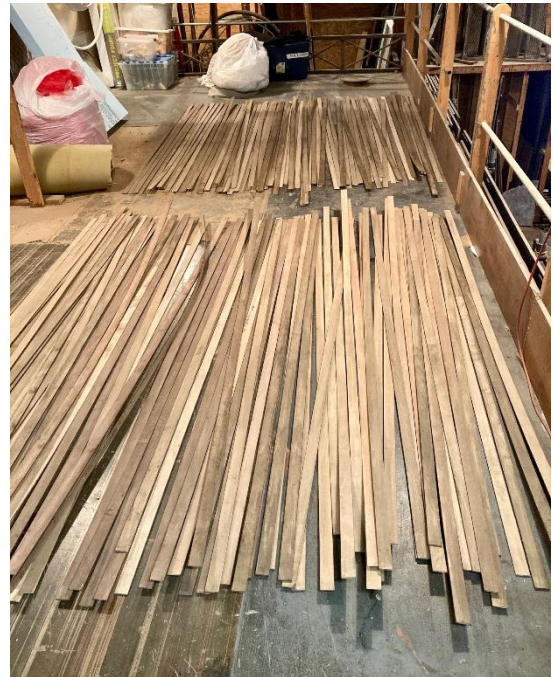
Figure 65: The slats of lath drying after staining. 2021, Tulane University.
