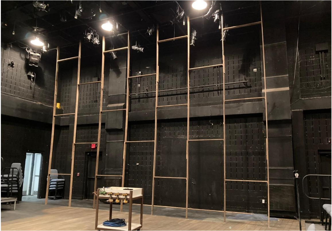
Figure 70: Framing for the upstage wall is installed. 2021, Tulane University.
