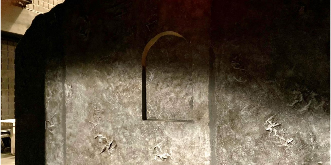
Figure 77: The alcove is cut out of the flat and plastered. 2021, Tulane University.
